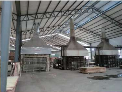
FF Plywood Plant
