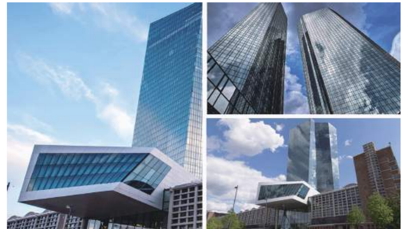
Project : European Central Bank Configuration: 5mm Clear +1.52mm PVB+6Low–E+16 A+5mm Clear +1.52mm PVB+5mm Clear Glass Location: Germany
