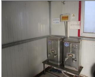
Photo of the sanitary facilities Drinking water.JPG
